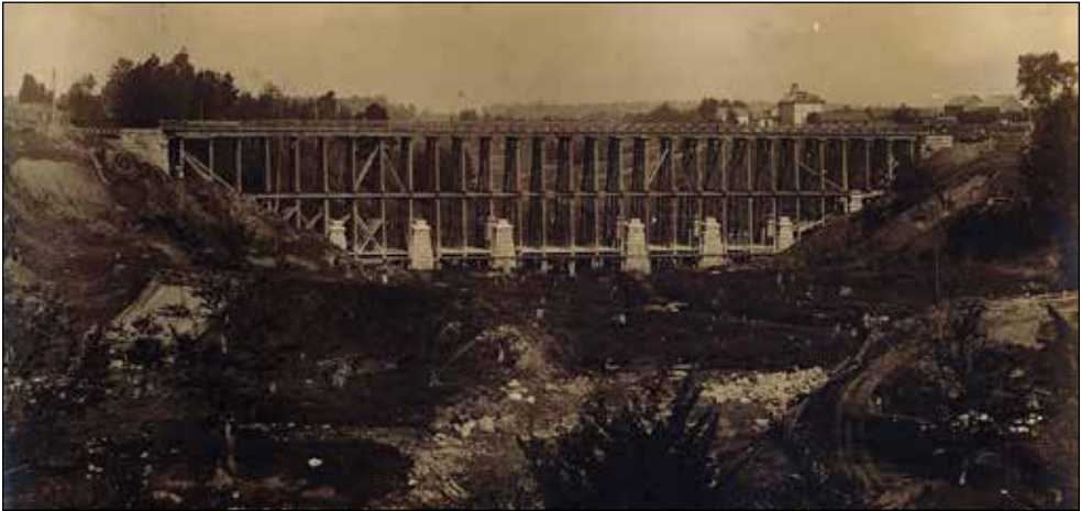
This photo from the 1870s shows the first bridge of the Great Western Railway being built to traverse Stoney Creek in what is now Participark. That original bridge was replaced by the current one in 1888. Note that the cement support pillars remained between the two structures, and will still be in use with the new bridge.
