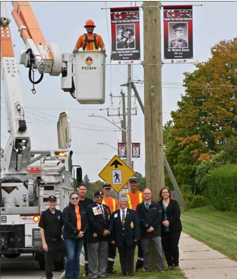
BANNER INSTALLATION COMPLETED (JEFF HELSDON PHOTO) Some of the partners responsible for the banners on Quarterline Road gathered with the completion of the installation of the banners. Left to right are: Frank Moore, Tillsonburg Military History Club; Sarah Jackson, Tillsonburg Hydro (THI) hydro ops coordinator; Kyle Jacob, THI linesman; Tom Brown CD, Tillsonburg Legion president; Kurt Hussey, THI linesman; Diane Hodges, Legion past-president; Grant Yarmie, THI linesman; Michael DeJong, THI finance manager; Niki Rogers, THI billing coordinator and THI linesman Ryan Fitch in the bucket.
