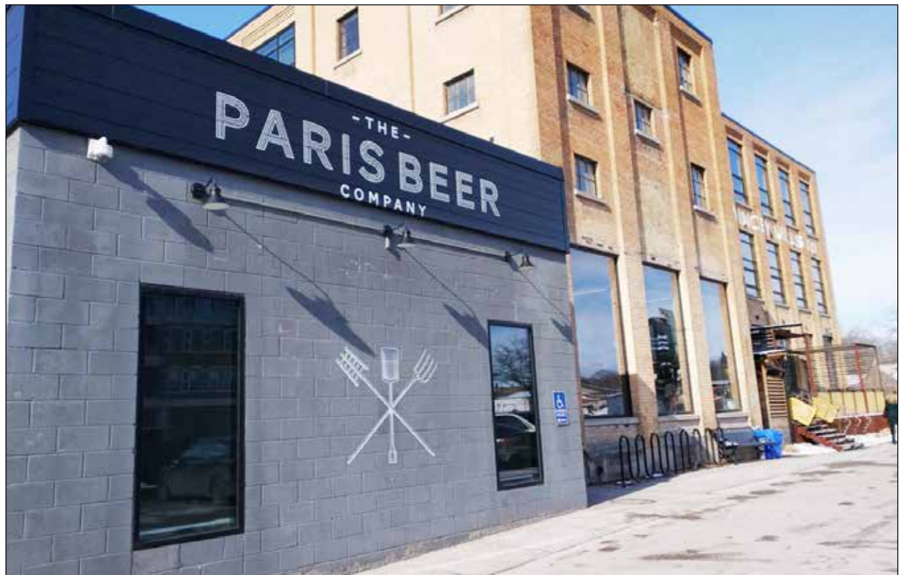
The Paris Beer Company brewery occupies a former garage at the back of the Wincey Mills in the Paris tourist area.
