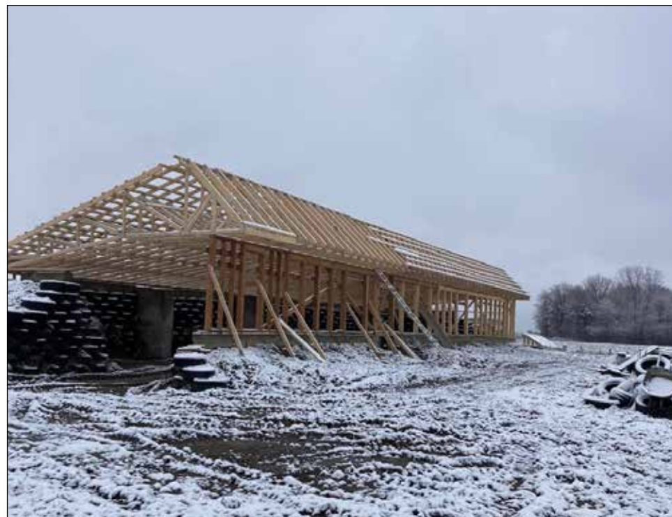
View of the newly roughed-in earthship and the north side berm before walls and windows.
