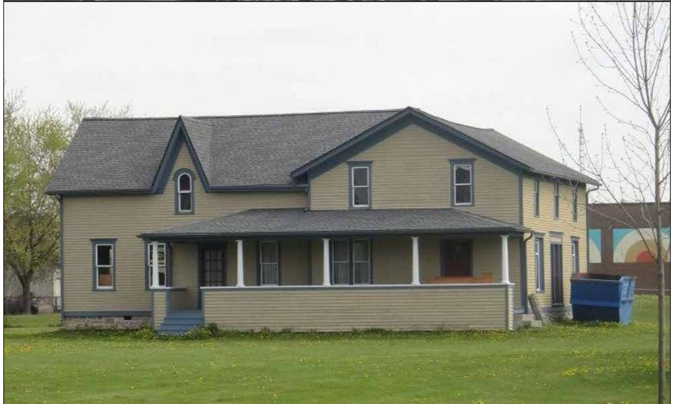
Eight years after a fire brought renovation efforts to the Minor House to a screeching halt, the Marshville Heritage Society is once again hoping to reopen the historic home to the public, and is seeking financial support to rebuild the 19th-century house. ~ Marshville Heritage Society photo
