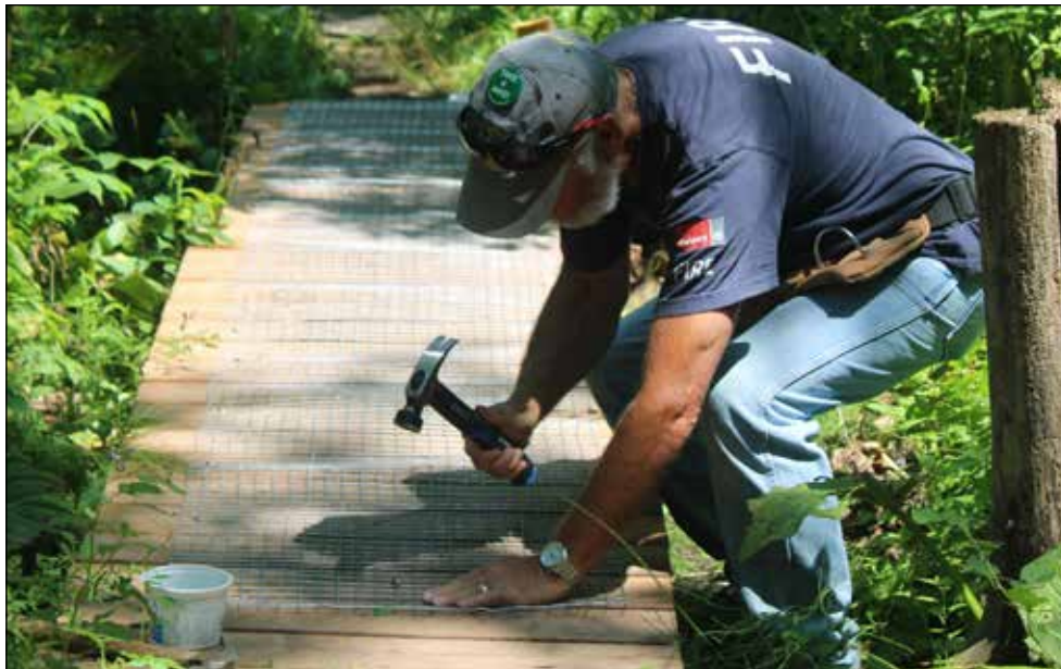
Cam Whiting installing some of the wire mesh.
