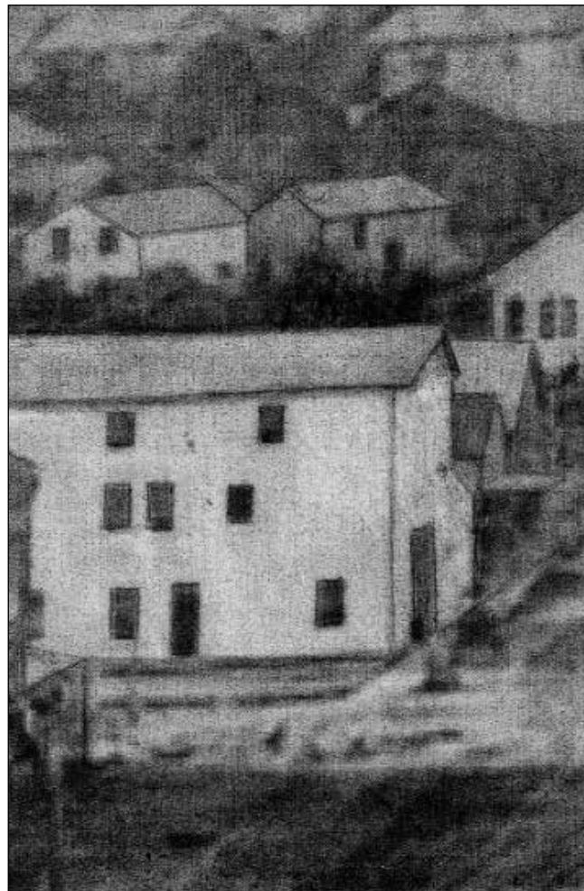
Here is a close up of the original Bradford Hotel
