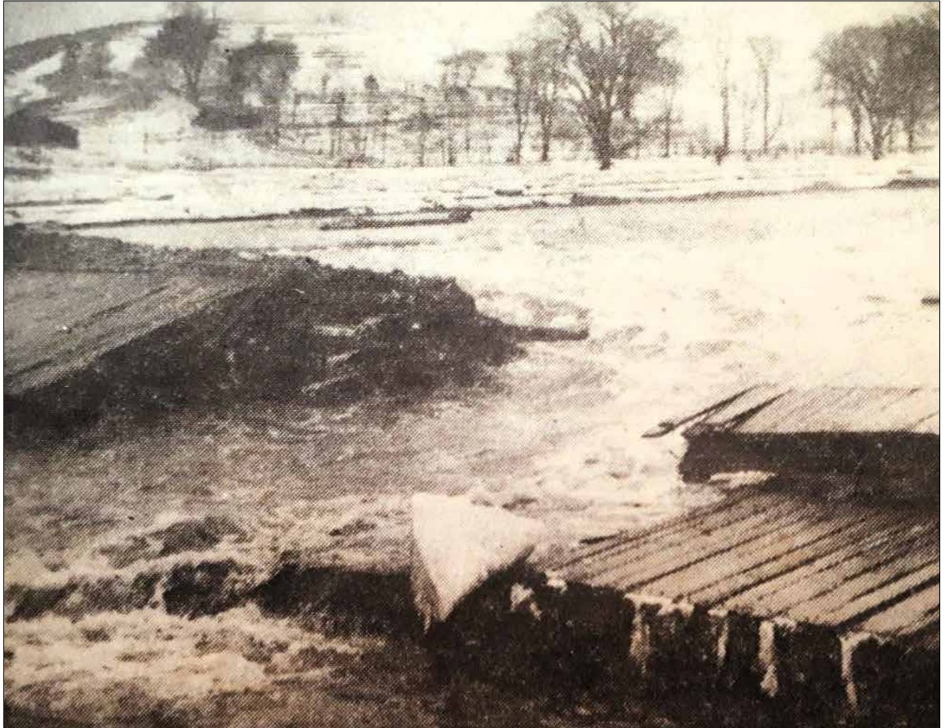
The oldest dam in Paris and first to be built on the Nith River, was breached by rain-swollen torrents from Hurricane Hazel. Within an hour, force of the water had cut a new course for the river leaving the Paris Wincey Mills without waterpower. Mill officials did not repair the structure but decided to switch to hydro electricity to power their machinery.
