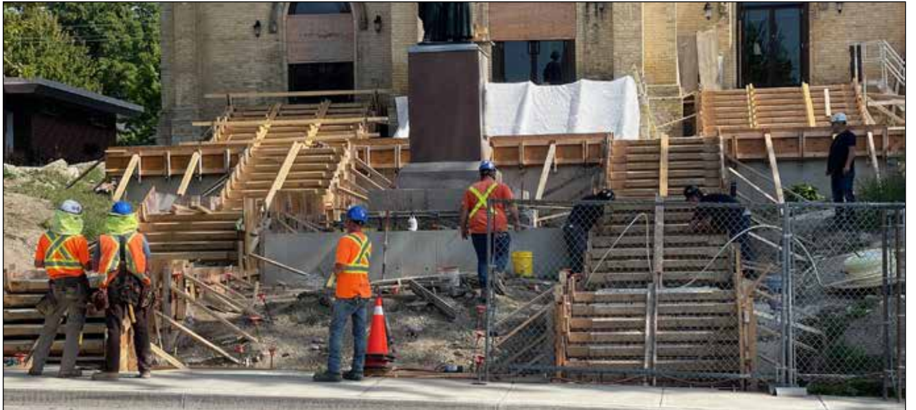
Work continues on the steps leading to St. Joseph's Catholic Church on Huron Street this week. With good weather, contractors expect the project to be complete in October or November.
