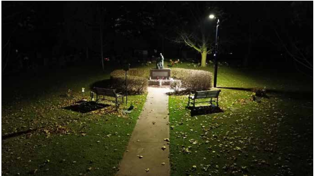
Solar-powered lighting illuminates a memorial at Holy Cross Cemetery, part of a new off-grid security system installed by Brant Municipal Enterprises to help deter vandalism while preserving the peaceful nature of the grounds.
