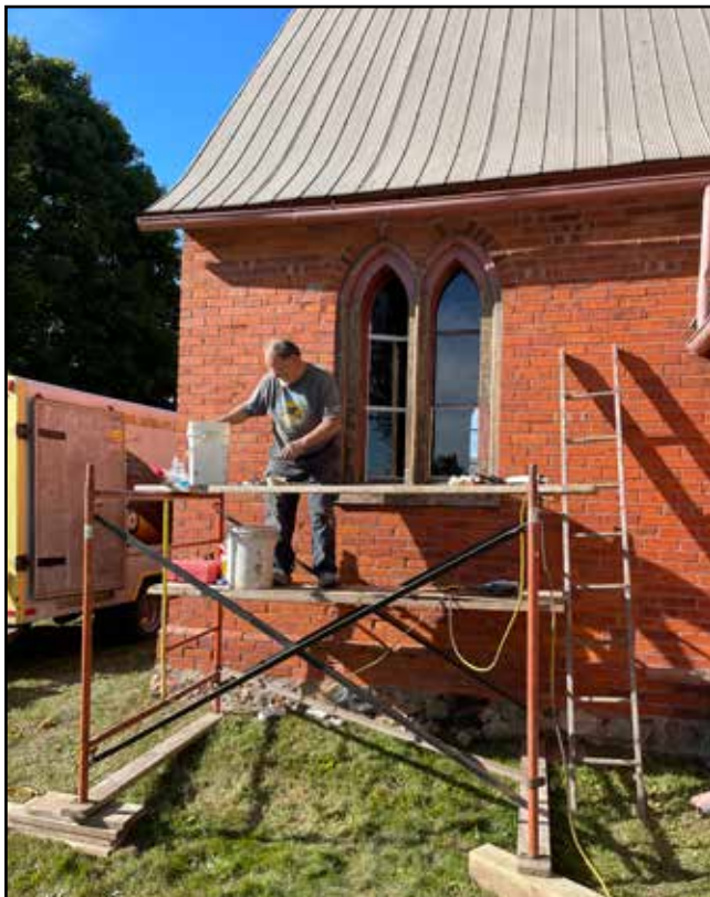
(GARY WEST PHOTOS) Carl Clayton repairs windows and frames on the south side of Trinity Anglican Church, two miles south of Tavistock, last week in the warm sunshine.
