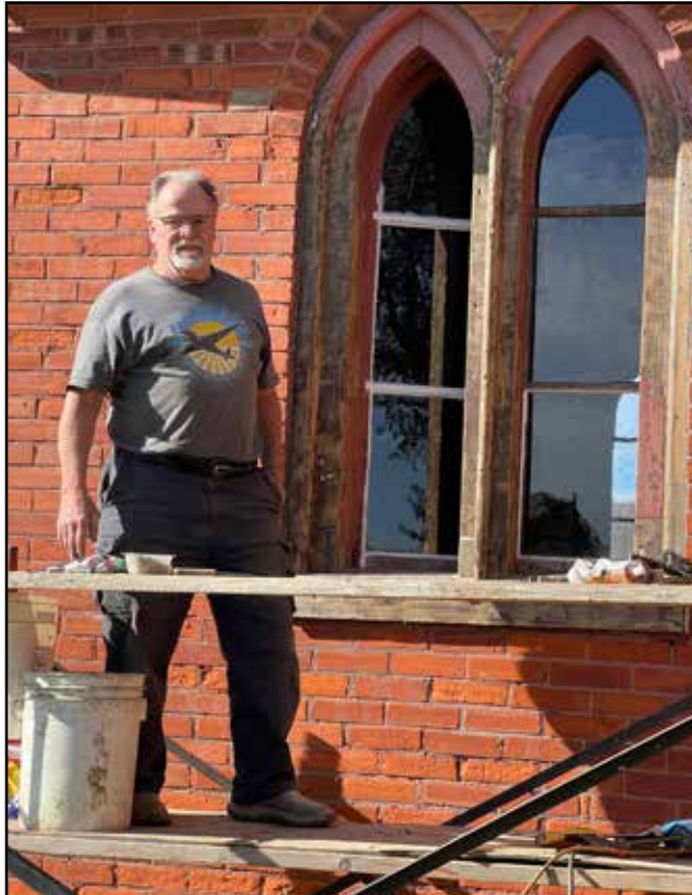
Carl Clayton pauses to share some of the church's history, noting it is approaching its 200th anniversary since construction in 1847.
