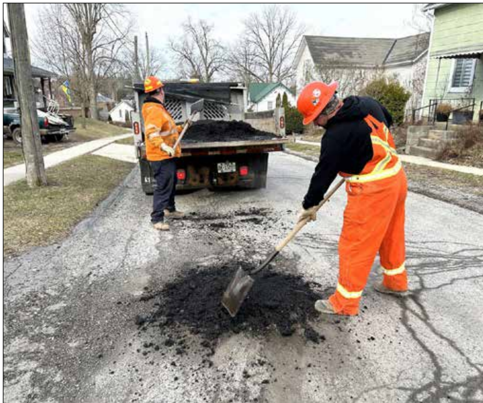
Road maintenance workers with Norfolk County fill in a pothole on Temperance Street in Waterford on Wednesday.
