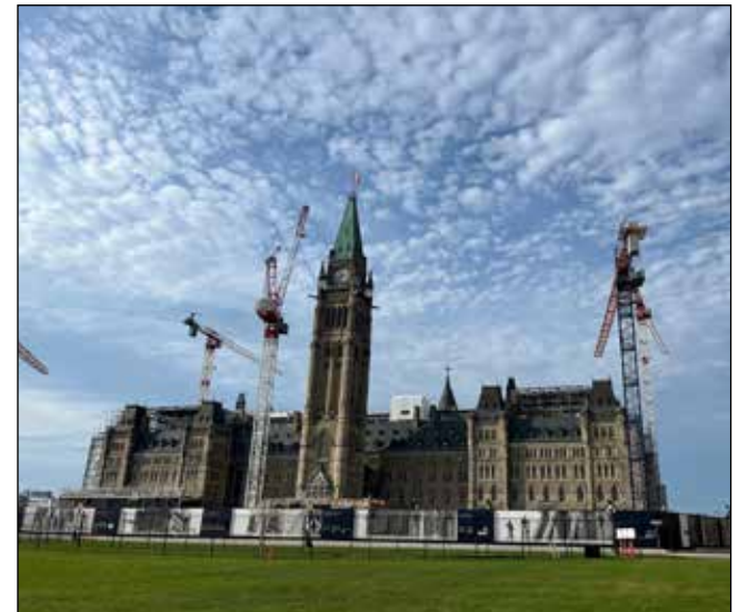
Parliament's Centre Block remains hidden behind walls and topped by construction cranes in a restoration project with no end in sight!
