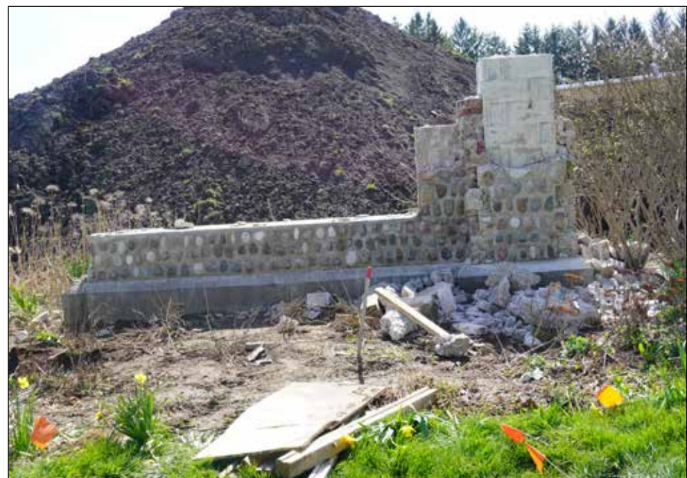
Pictured is the Thorndale gateway sign after the key components were dismantled on Saturday, April 25.
