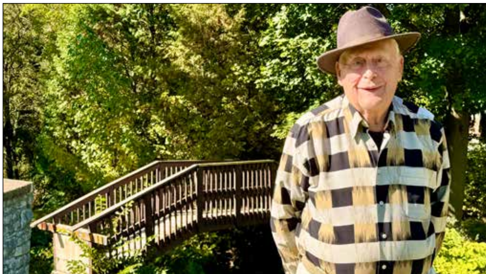
Reg White, a member of the informal Friends of the Shakespearean Gardens group, stands in front of the iconic bridge to the island. It is slated to be removed due to deterioration and non-compliance with the Accessibility for Ontarians with Disabilities Act, as announced to council on June 11.
