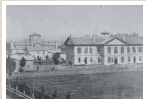
Court House Square photograph, 1865, Oxford County Archives
