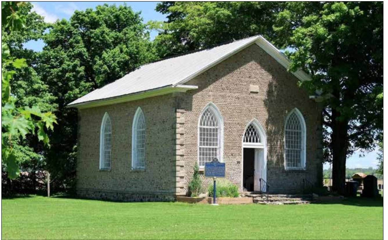
The historic Paris Plains Church, built in 1845, remains one of the finest examples of cobblestone architecture in the region. A public meeting on June 15 will help determine the future of the landmark as caretaker Ray Perriman seeks community support to preserve the church and adjacent Maus School for future generations.
