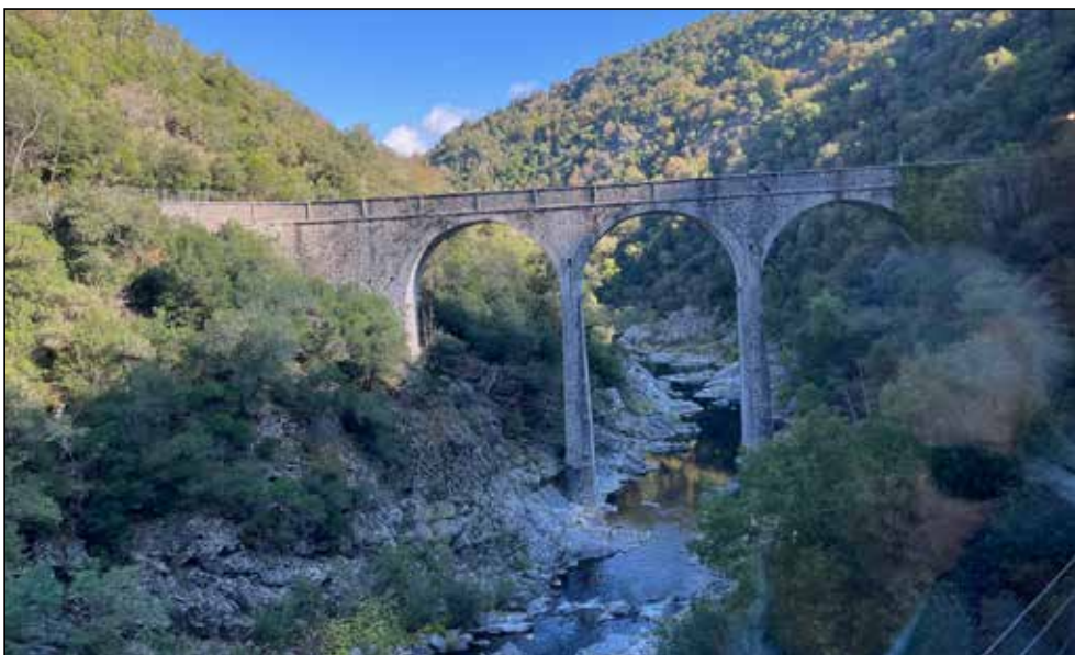
An aqueduct in the Doux Gorge.
