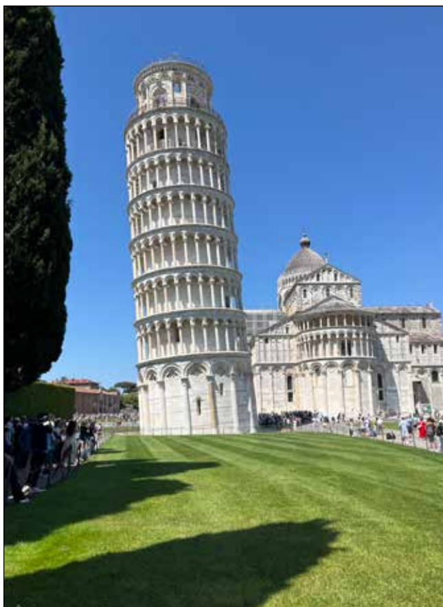
The tilt of the Leaning Tower of Pisa is clearly evident, caused by unstable subsoil.
