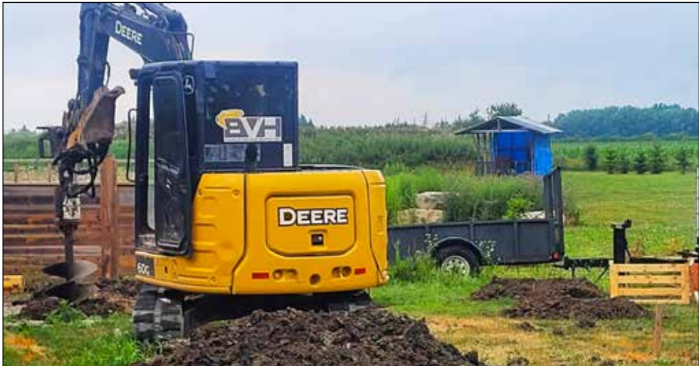
Construction of a tiny home starts at a St. Marys residence. Teahen Construction has been the lead local contractor involved with the build.
